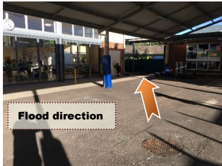
Plate 4 Floodway southern view
