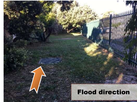
Plate 2 Southern floodway looking east
